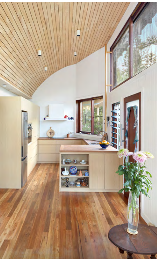
↑ Floors are FSC-certified engineered spotted gum boards. The kitchen benchtop is also of spotted gum, reclaimed from another of the builder's projects.
